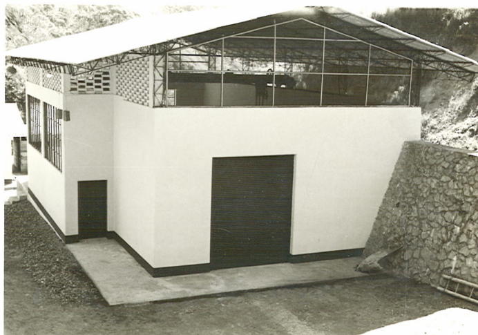
Figure 12 Outside View of Powerhouse
